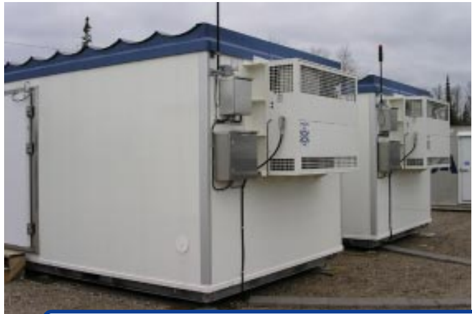
6 special units delivered to GM® cold weather development center in Kapuskasing, Ontario, Canada. These units can pull down to -45° C room temperature.
